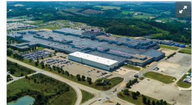
Located at RIDC's Westmoreland Innovation Center, Intervala connects Pittsburgh's innovation ecosystem to real-world manufacturing.
